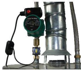
Hot Water Line Installation
