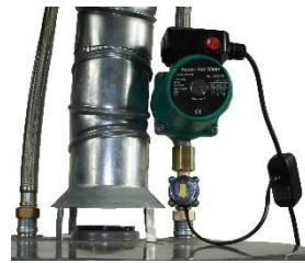
Cold Water Line Installation
